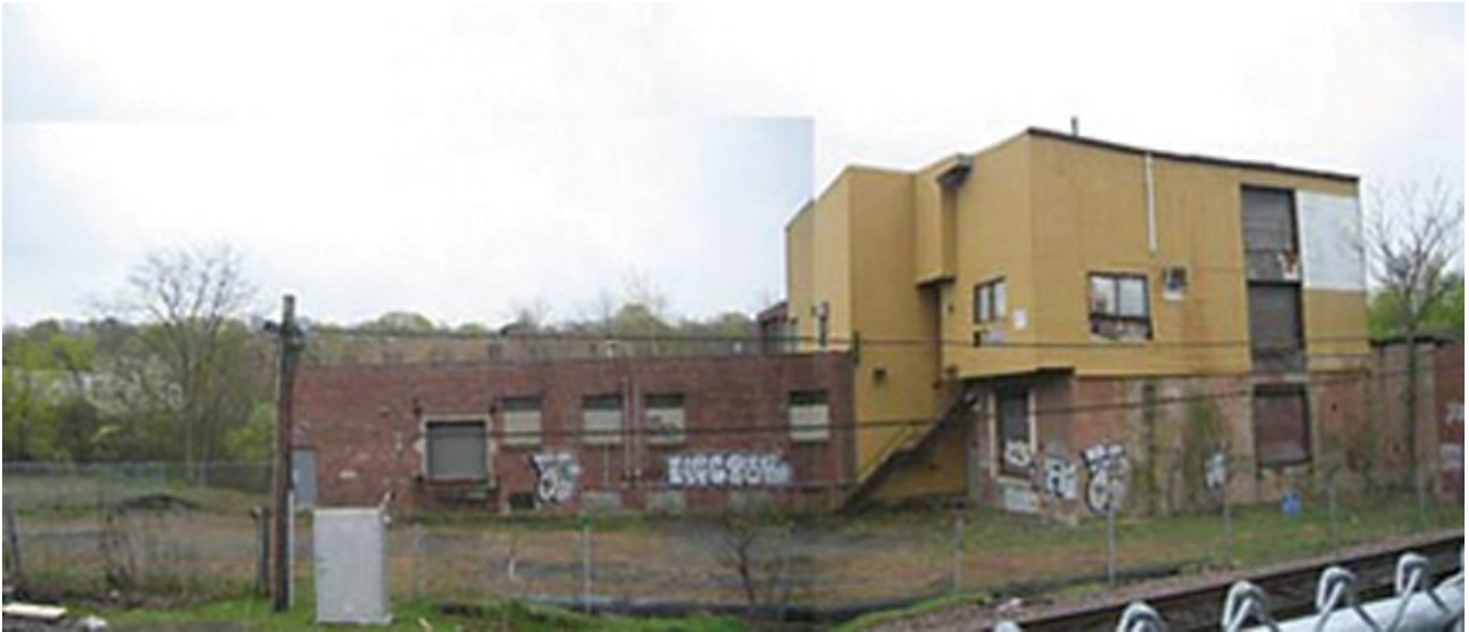
The Lewis Chemical building on the bank of the Neponset River before being torn down in 2013. Lewis Chemical operated from 1963 to 1983 and was cited for a number of environmental violations. Photo Courtesy http://www.swbcdc.org
